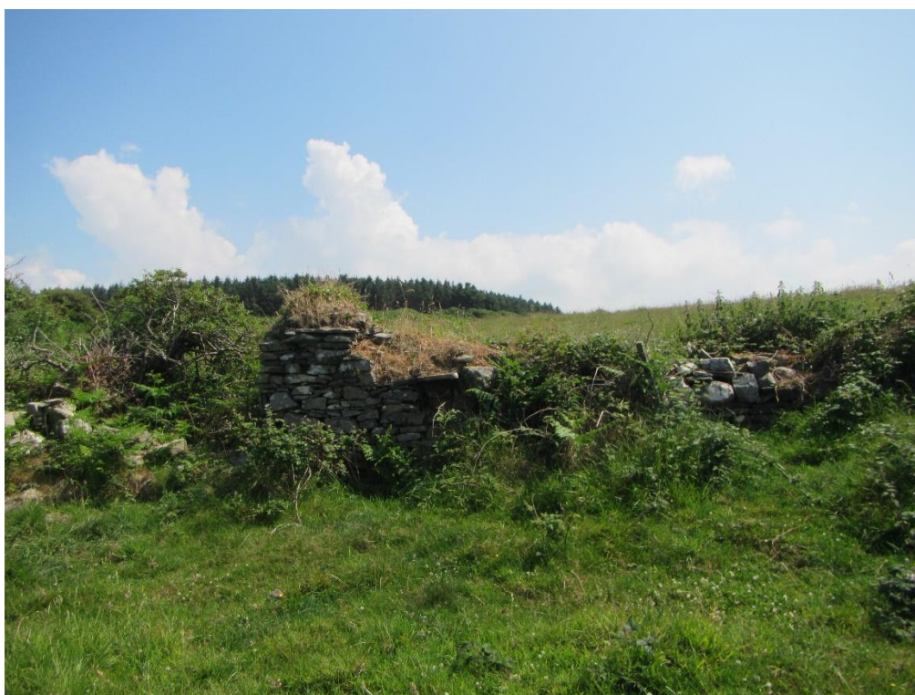
Photograph 12.8 CHS15 Structure within the Proposed Development.
