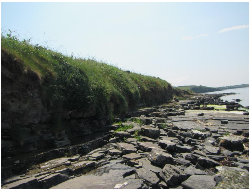
Photograph 12.9 The proposed location of the Stormwater Outfall.
