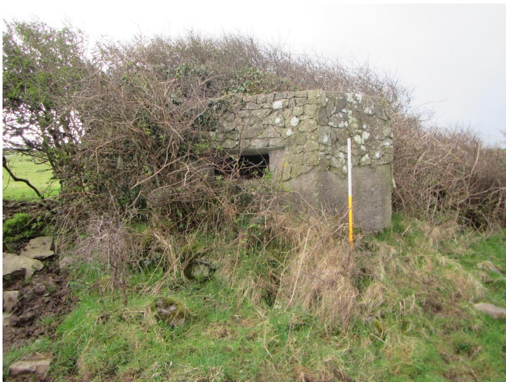
Photograph 12.7 CHS7 Gun Emplacement within the Proposed Development.
